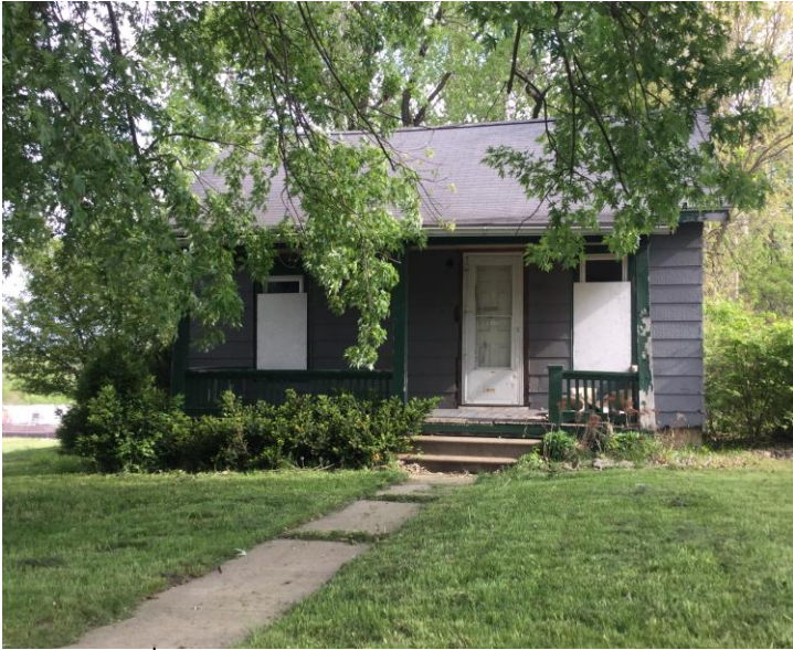
1372 22 nd Ave SW GPN #14322-81017-00000 Photo taken by DS on 5/8/2017
